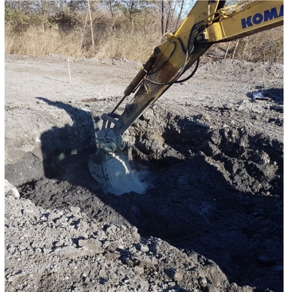
PC addition and soil mixing
