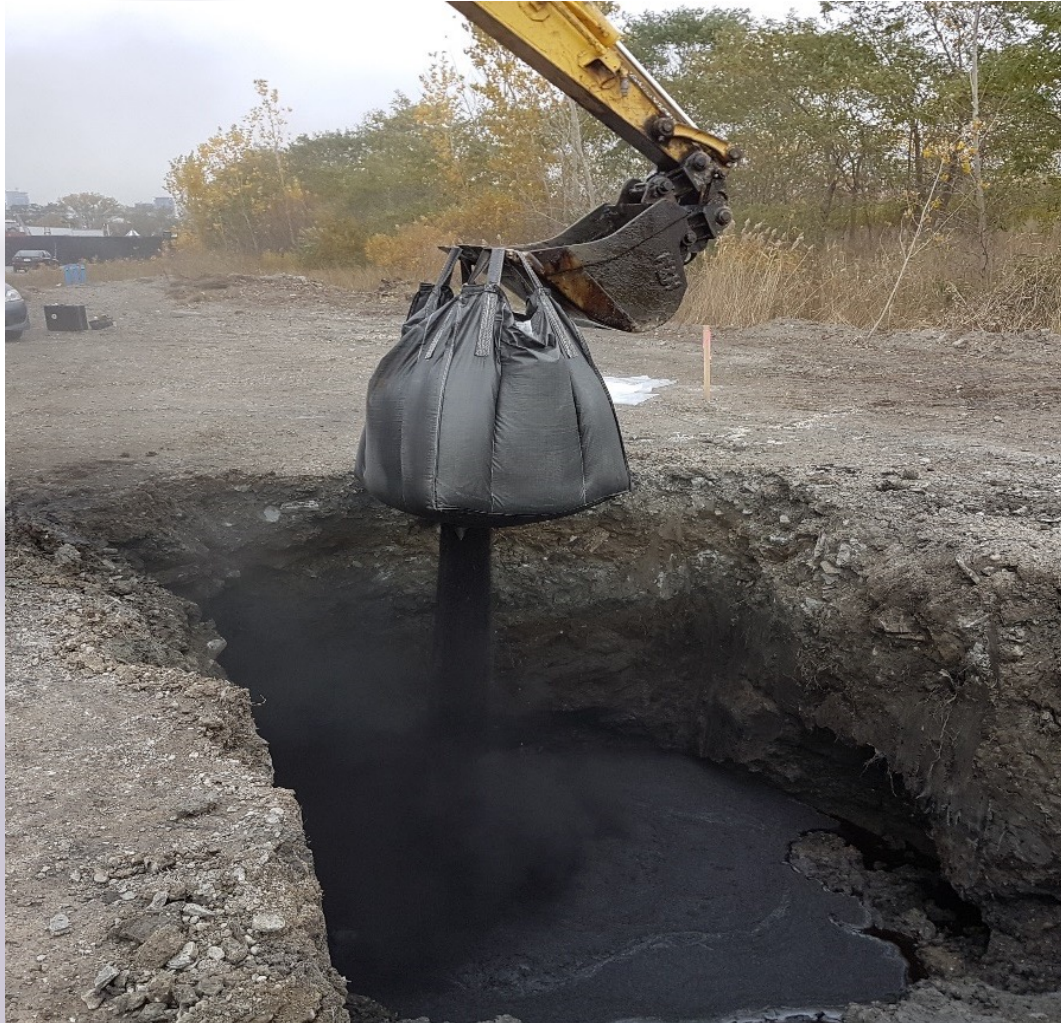
GAC addition and soil mixing
