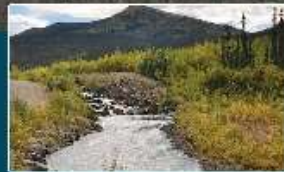
2. Rose Creek Diversion
