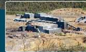
5. Mill Area - Faro Water Treatment Plant
