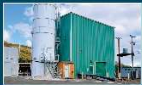
13. Vangorda Water Treatment Plant
