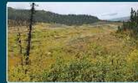
10. Fresh Water Supply Dam & Reservoir
