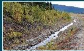
8. Faro Creek Diversion
