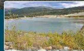
4. Cross Valley Pond & Dam
