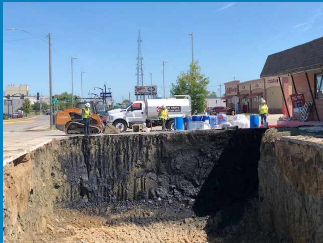
Excavation polish with PetroFix
