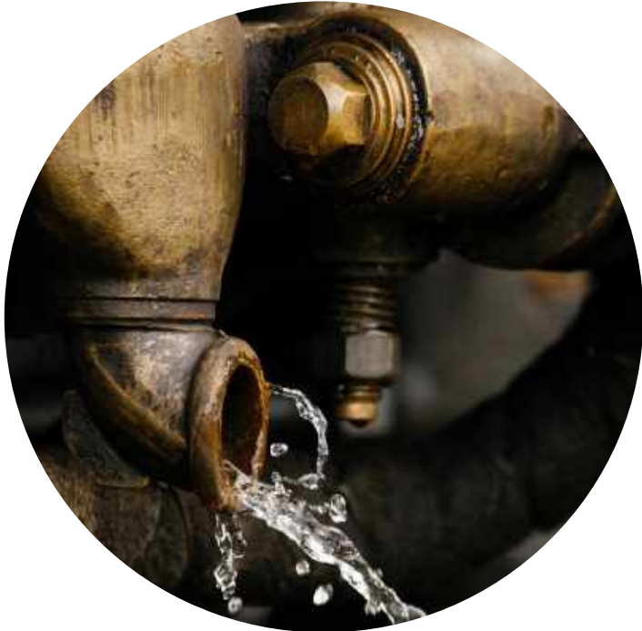
Ground Water Treatment Pumping & Conveyance
